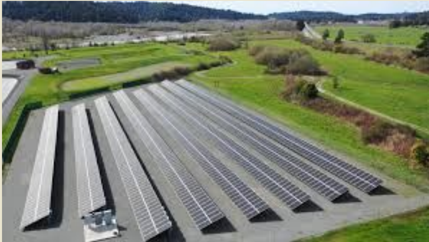
Blue Lake Rancheria Microgrid (source: Blue Lake Rancheria)
